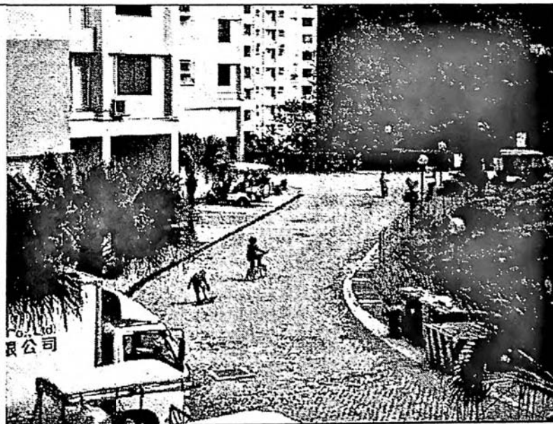
Section 3 of Parkvale Drive – "The Passageway". The far end of the pedestrian pavement is from where the proposed extension of Parkvale Drive will start.
