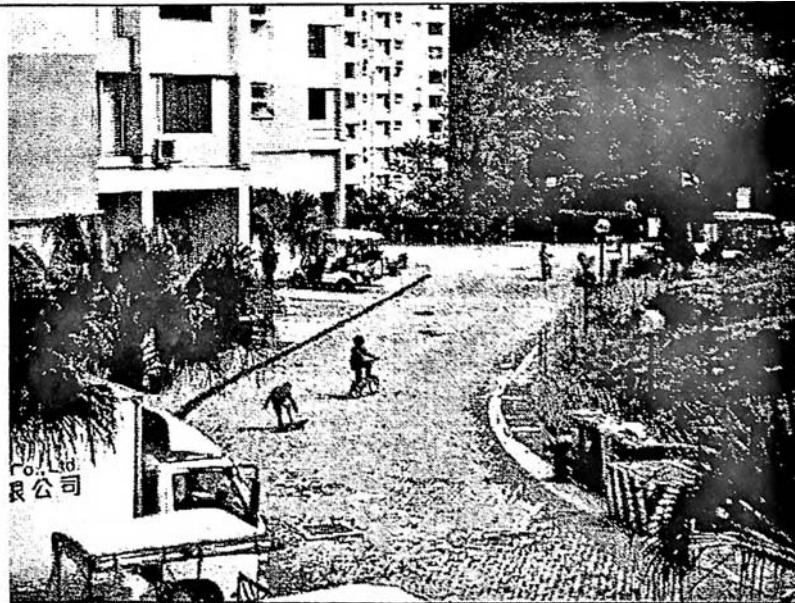
Section 3 of Parkvale Drive – "The Passageway". The far end of the pedestrian pavement is from where the proposed extension of Parkvale Drive will start.
